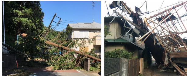
Power outage damage caused by huge typhoon No. 15 in 2019 Source: METI
