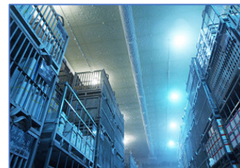
Freezing storage facility
