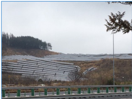
Solar Power generation
