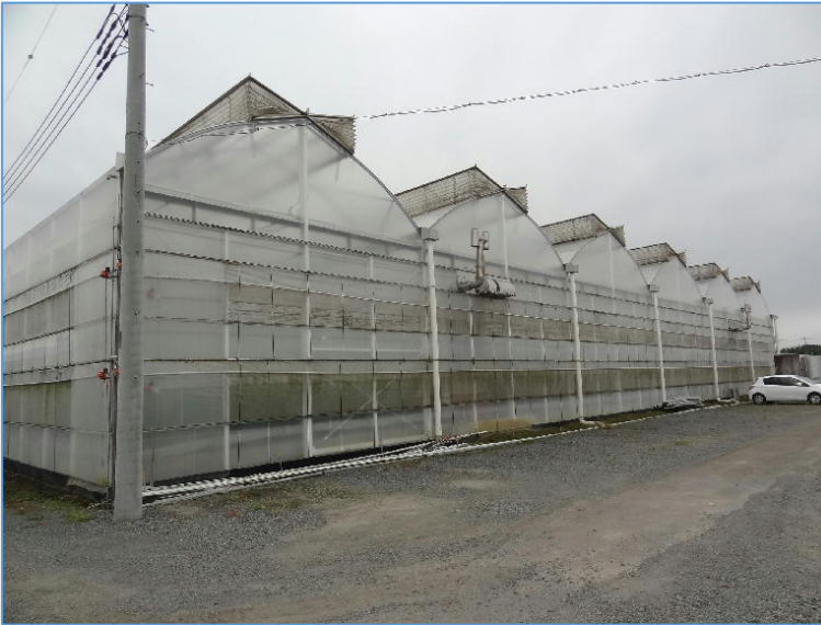
Exterior of demonstration greenhouse
